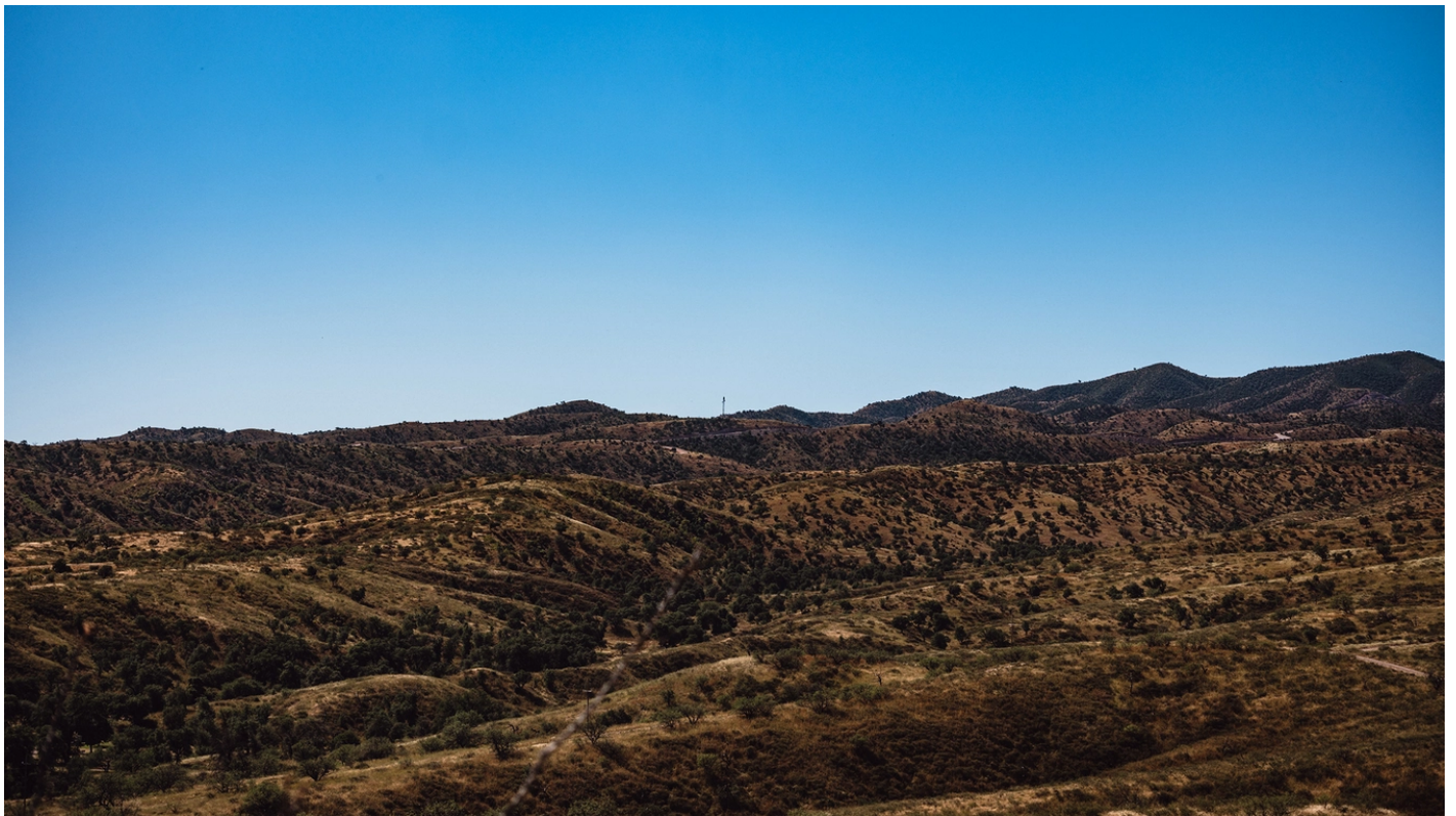
An Elbit Systems surveillance tower in Sasabe, Ariz.
